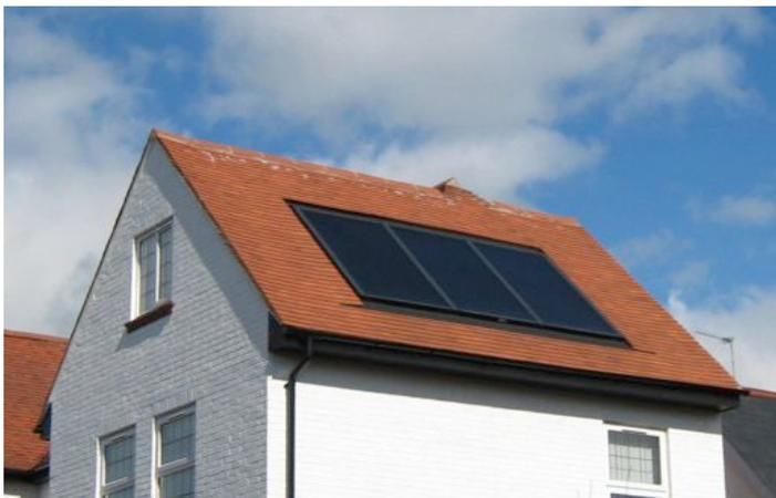
*These panels are evacuated tubes behind glass (Vaillant)*
